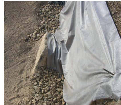
Figure 71 Drain installé.
